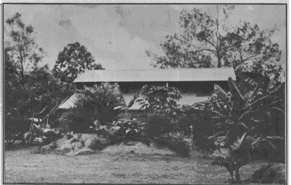
Australia: The newly constructed 'Bhakti Centre' with Prasad hall downstairs, and office and accommodation upstairs.
